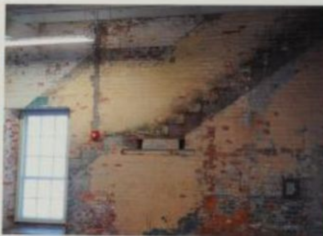
ABOVE AND OPPOSITE show structure and existing finishes in the galleries.
