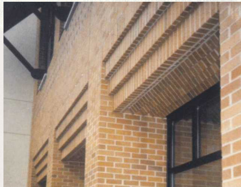
Figure 1. Lintel system has a concealed steel spine that spans the opening. The spine supports cored brick laid in soldier courses to create an all-masonry soffit.
