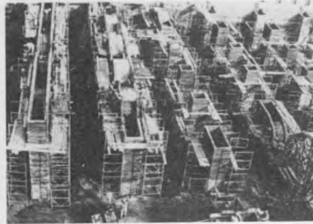
Fig. 86: View during construction showing the "clay pipes" Rafael Moneo: Museo de Arte Romano, Mérida (E), 1986
