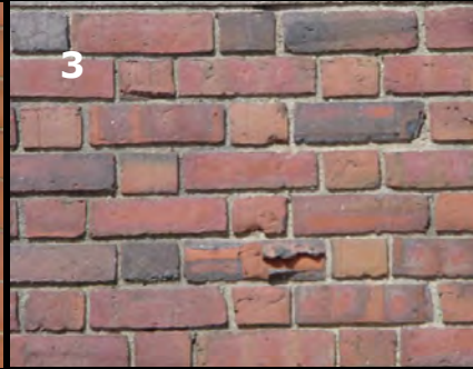
Running Bond consists entirely of stretchers
