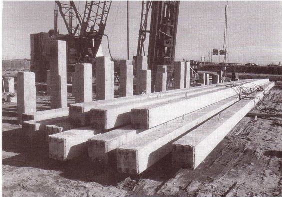
FIGURE 2.43 Precast, prestressed concrete piles. Lifting loops are cast into the sides of the piles as crane attachments for hoisting them into a vertical position.
