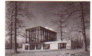
Fig. 57: Substructure and superstructure as structurally independent constructions with the same use (residential)
